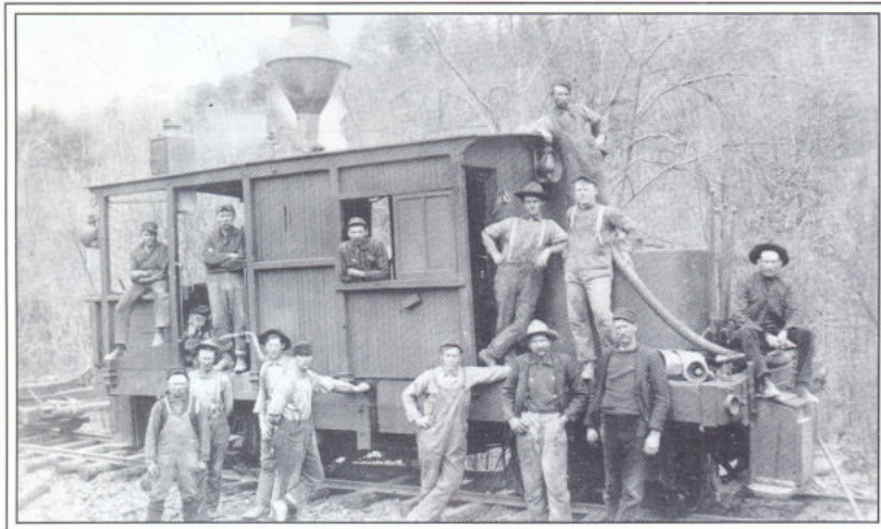
This vertical-boilered Class A Climax has a fully enclosed cab, a round water tank, a large old-style headlight, and a tall smokestack. Note the siphon tube on the water tank for taking water from track-side streams. Photo, collection of Benjamin F.G. Kline, Jr.
